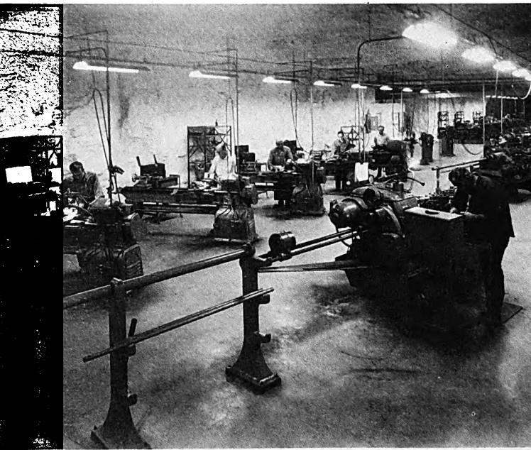
A FACTORY IN LIMESTONE — Workers make precision measuring instruments in this underground 140,000-square-foot plant carved out of solid limestone by the Brunson Instrument Company in Kansas City, Missouri.
